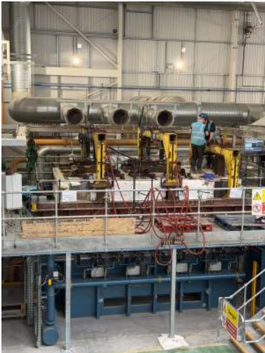
Setting Up Furnace and Loading Frames
